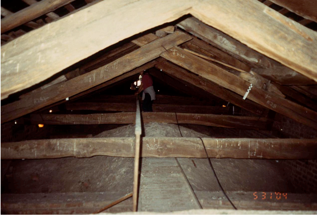
Figure 14. Viboldone, abbey church (completed 1348). Nave vault from above. Although the roof is a replacement, the main cross beams are original, almost touching the tops of the vaults.
