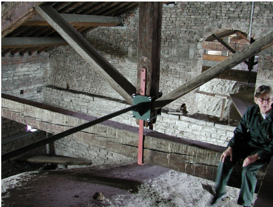
Figure 13. Santa Maria Novella. Above nave vaults, showing transverse wall between bays.
