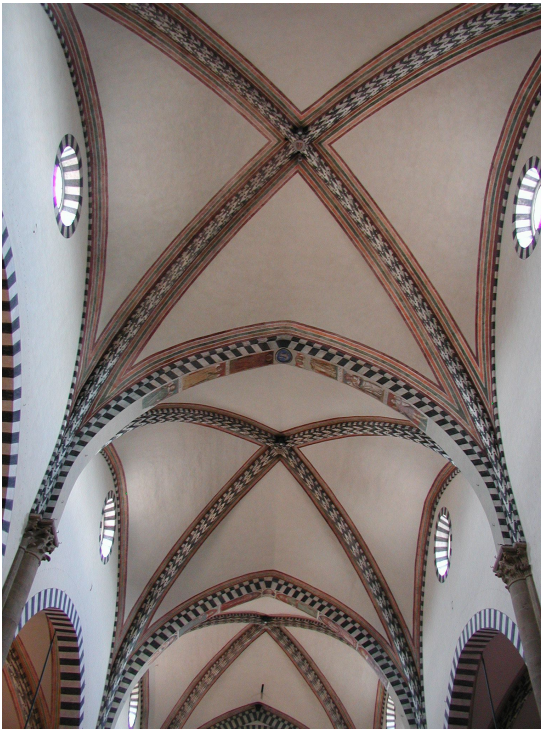
Figure 10. Santa Maria Novella, nave vaults over square bays
